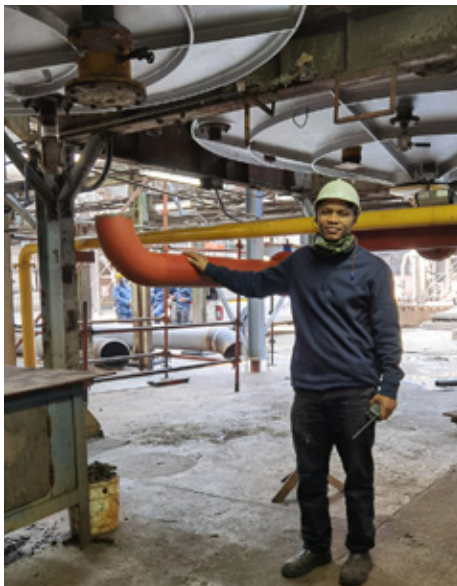
Cebo Khumalo, Plant Engineer, seen here at the soon-to-be revived evaporators
